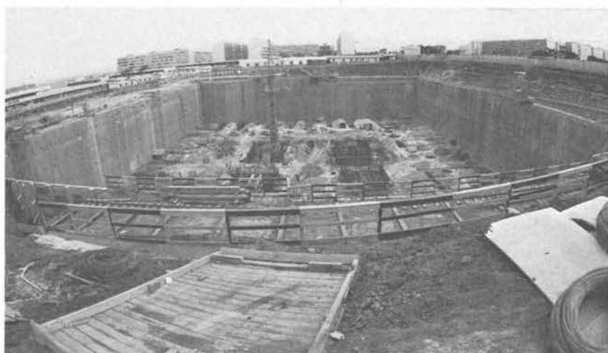
Fig. 1. — Photograph of the excavation and the anchored wall.
