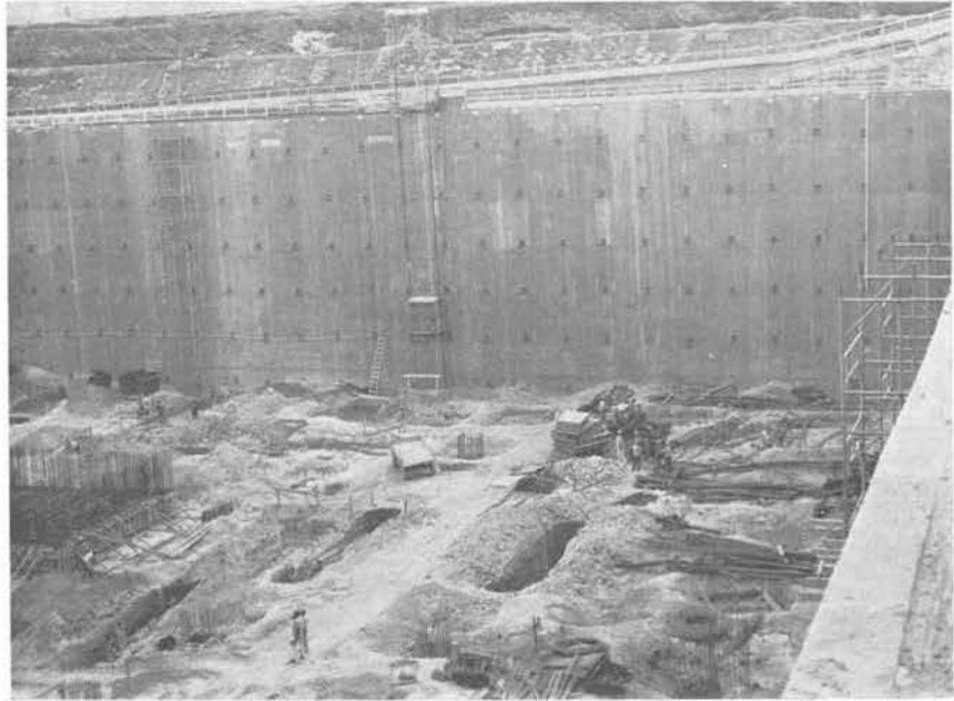
Fig. 2. — Photograph of the excavation and the anchored wall.
