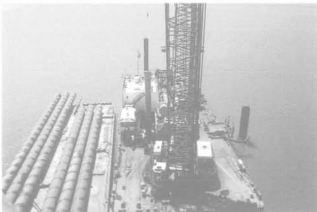
FIG. 6 Barge de battage. Pile driving barge.
