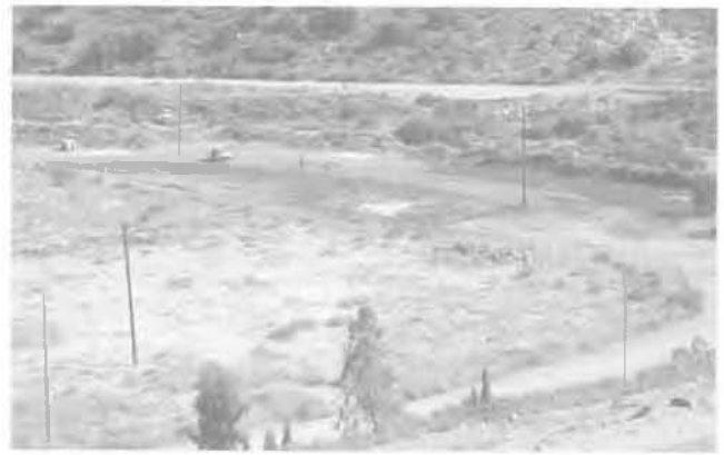
FIG. 6 Le remblai routier terminé (2003). The road embankment completed (2003).
